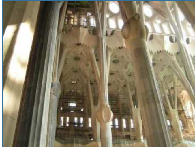
The forest of branching columns that holds up the vaults.
