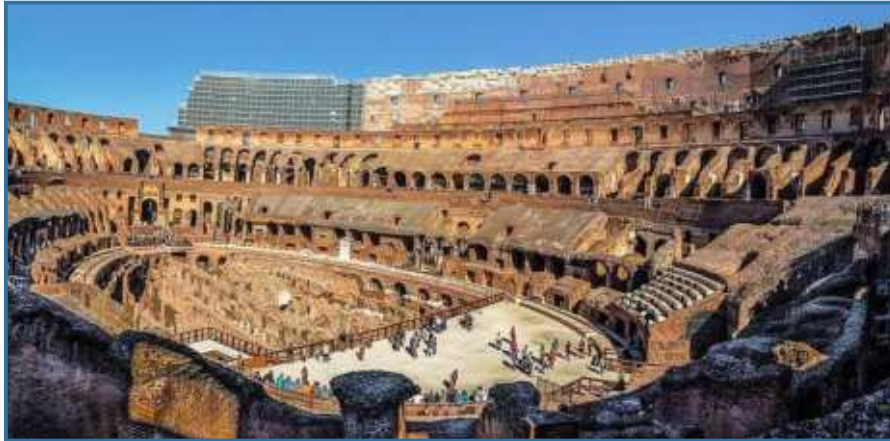
The hypogeum: the underground chambers beneath the Colosseum's arena.
